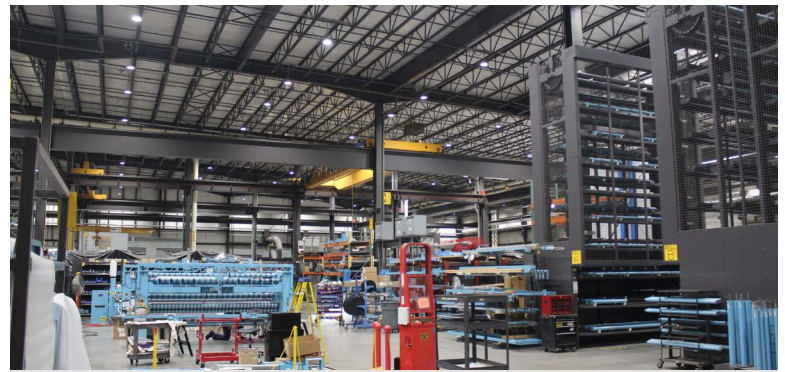
Dialight Vigilant® LED High Bay fixtures at the G.A. Braun facility.
